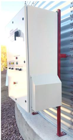
**Simple installation:** Site electrician supplies incoming power to the panel and connects it to the motor.
