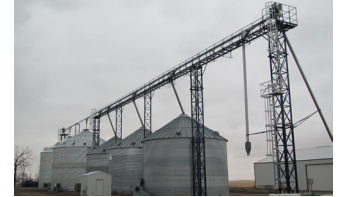
Sudenga tower and catwalk
