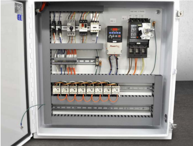
MOTOR CONTROL PANEL The motor control panel with VFD controls allows for each hopper to be set to an individual high and an individual low speed setting through the batching control panel.
